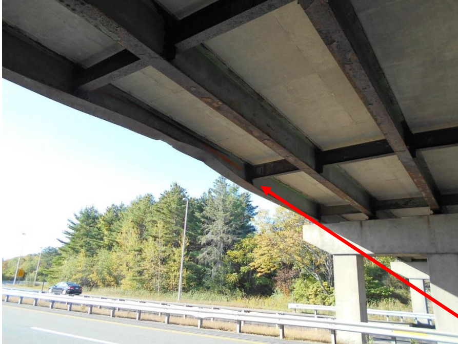
Bent diaphragm connection plate
